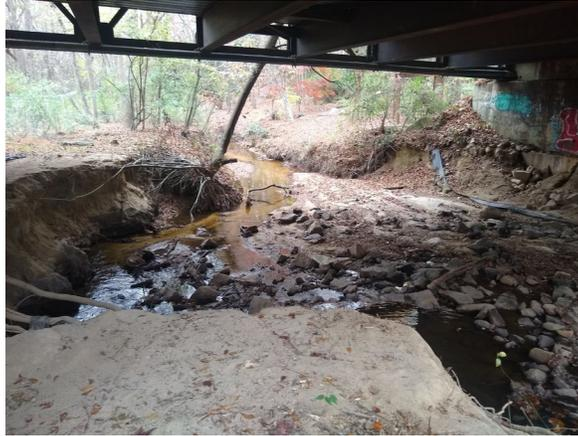
*Figure 11. Severe Erosion on Toms Creek*
